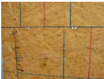
Figure 3. OSB Wall Construction
