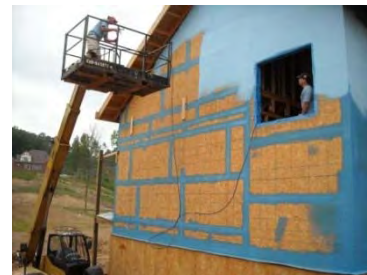
Figure 5. Spray Installation of Barriteck VP
