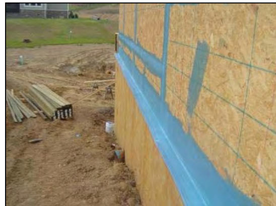
Figure 13. DCH Fabric Imbedded in Baritech VP as Base Wall Flashing
