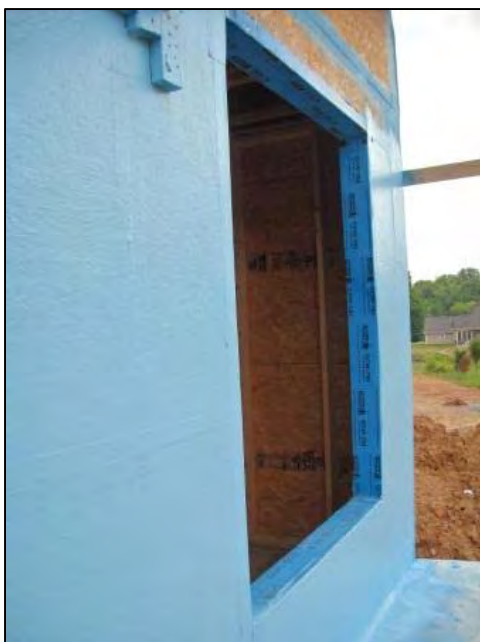
Figure 15. CCW-705 Self-Adhering Flashing in Window Opening
