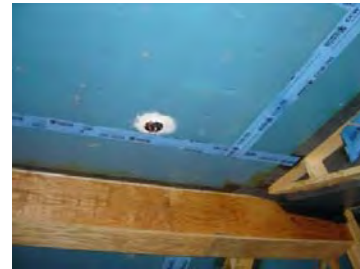
Figure 11. Ceiling Air Barrier, Joints Taped with CCW-705 or Barritape
