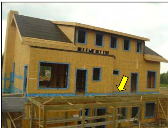
Figure 12. CCW-705 Self-Adhering Membrane Between Deck and Wall
