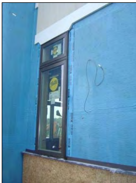
Figure 16. Window Installed in Opening
