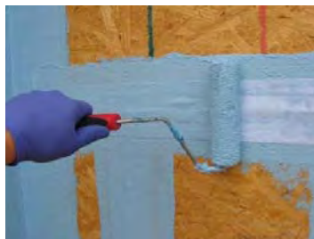
Figure 4. DCH Fabric Imbedded in Barriteck VP
