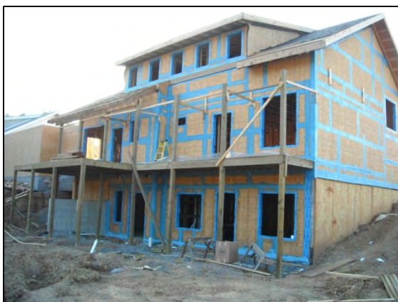
Figure 18. Overview - Detailing of Joints and Penetrations
