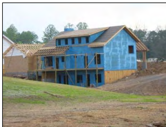
Figure 19. Full-Coverage of Exterior of the OVF test Home with Barritech VP Fluid-Applied Membrane
