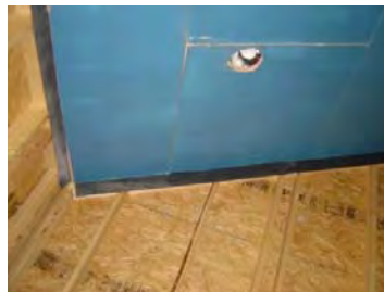
Figure 10. Foil-Faced Boards in Ceiling Coated with Barritech VP
