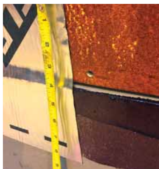
Peel & Stick Flashing Installed at Junction of Dissimilar Substrates. Substrates Prepped with Contact Adhesive (red)
