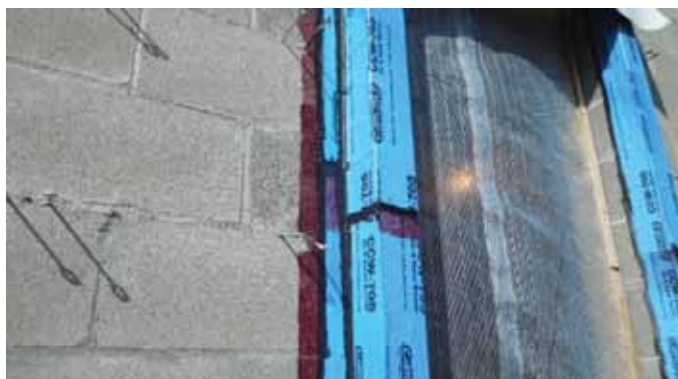
Peel & Stick Flashings with Termination Mastic at Edges – Ready for Liquid WRB
