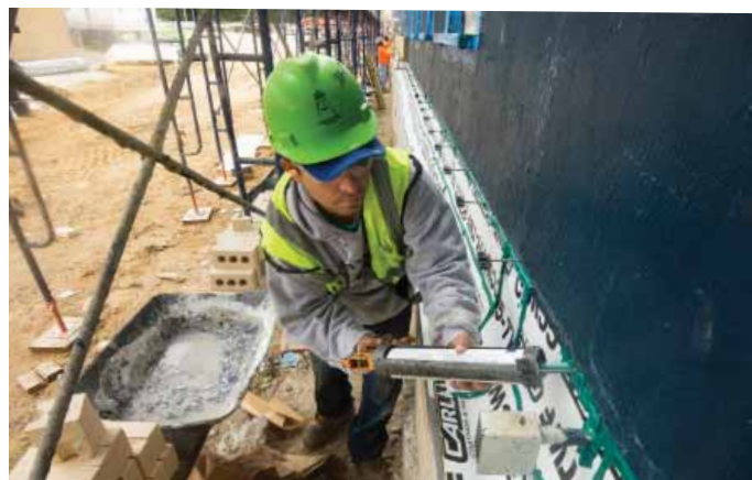
Peel & Stick Flashing applied after liquid WRB (Through Wall Flashing)
