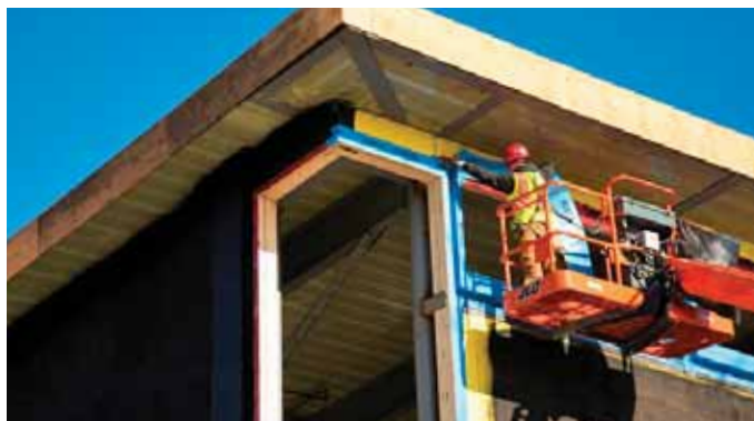
Peel & Stick Flashing Application in a Liquid WRB System on a Project
