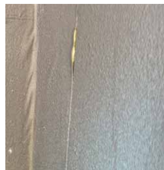
DON'T DO THIS...Peel & Stick Flashing Curl-Up Due to Missing Termination Mastic
