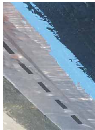
Peel and stick Flashing installed after Liquid WRB at Termination
