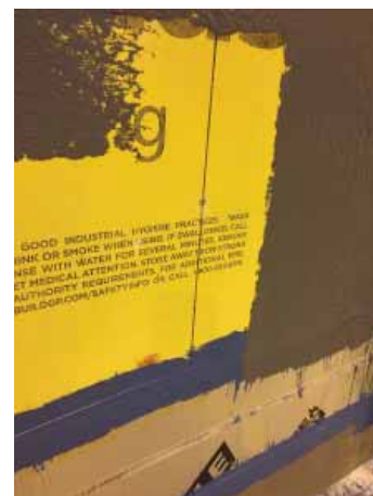
Liquid WRB Applied over Peel & Stick Flashing
