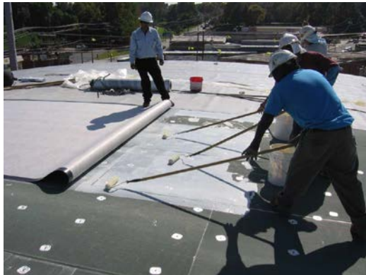
Felt-faced polyiso on roof
