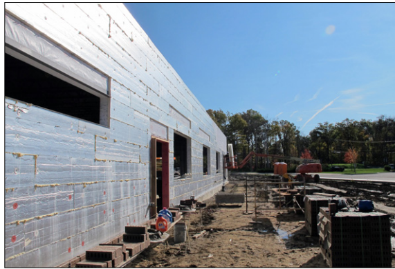
Foil-faced polyiso on wall
