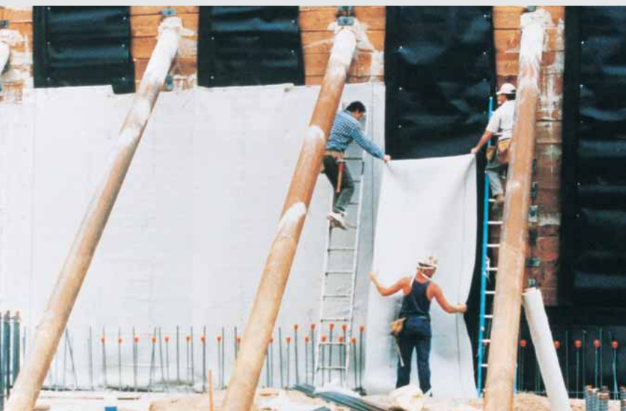
Soldier Pile Support with CCW MiraDRAIN and CCW MiraCLAY
