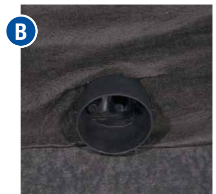
6" Sideout Connector covered with fabric
