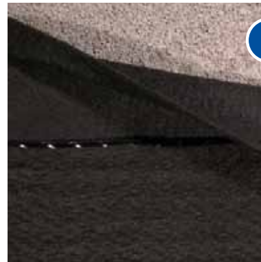
Cut approximately 3" (75 mm) of core leaving the geotextile fabric to overlap the adjacent panel. The fabric can be adhered with approved CCW adhesive. (Optional: Cover butted core with additional geotextile fabric.)
