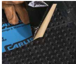
CCW MiraDRAIN joined in a "T" intersection with 4" CCW-705 or Aluma-Grip 701.
